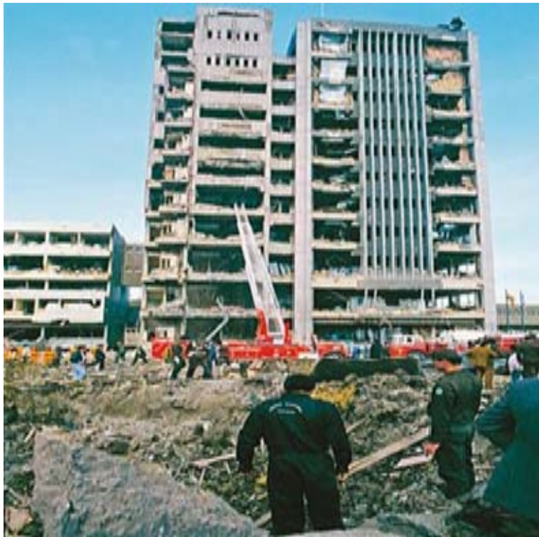
Figure 11. Departamento Administrativo de Seguridad (DAS) building in Bogota in 1989 after one of Pablo Escobar's bombs went off. DAS is equivalent to the United States Federal Bureau of Investigation. (From Bowden, 2001).
