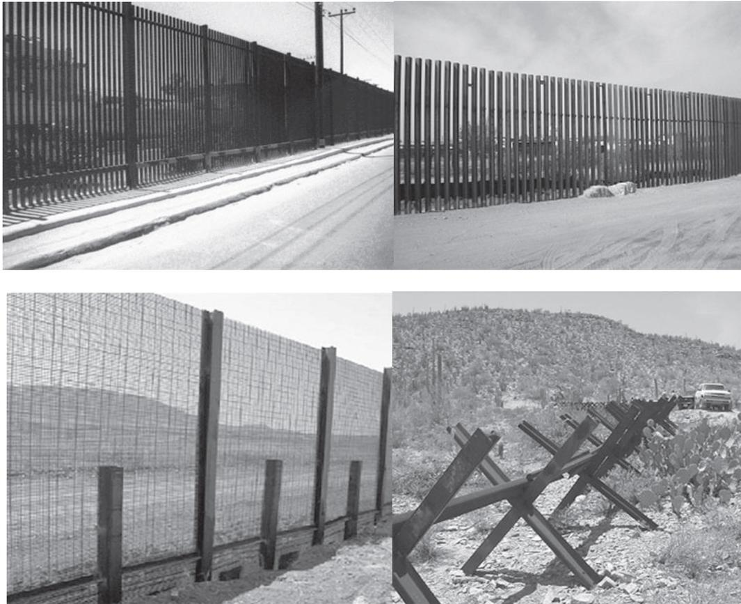
The Picket Fence (upper left), Bollard Fence (upper right) and Post & Rail with wire mesh (lower left) are examples of pedestrian fencing; the Normandy Vehicle Fence (lower right) is an example of vehicle fencing.
