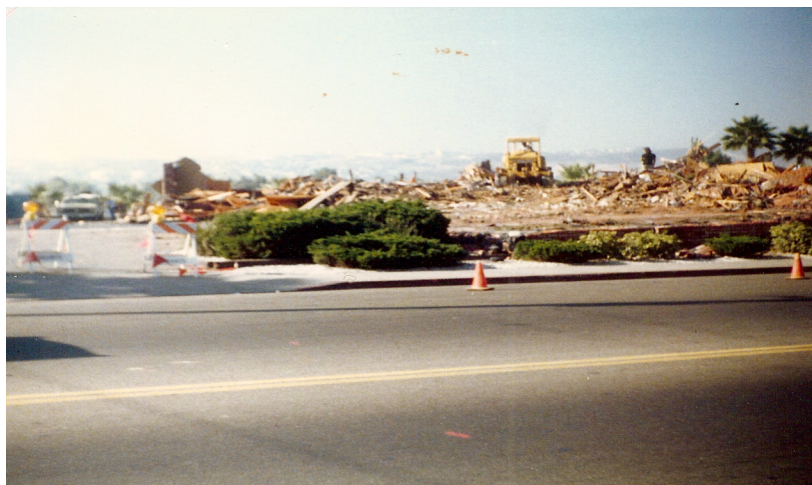
FIGURE 7: McDonalds site being razed. Photo courtesy of Consuelo Delgadillo
